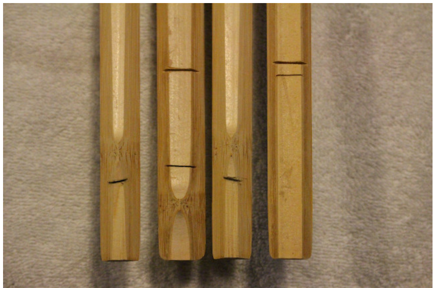
Figure 93: New grooves must be cut into the replacement slats.
